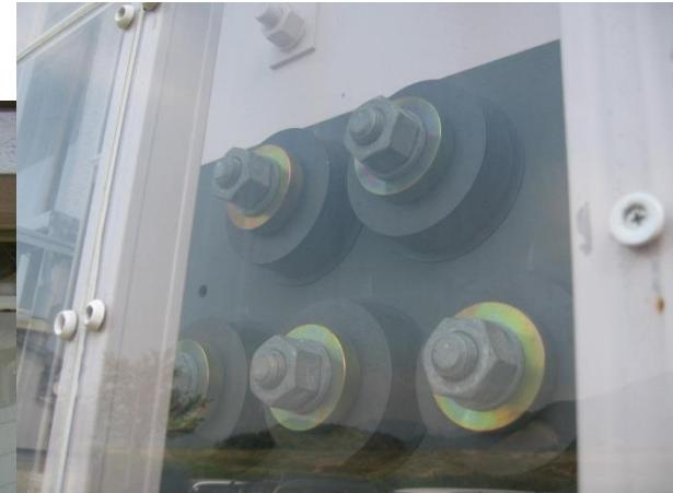
⑬ Friction damper can be seen from outside as appealing and visual checking after earthquakes.
