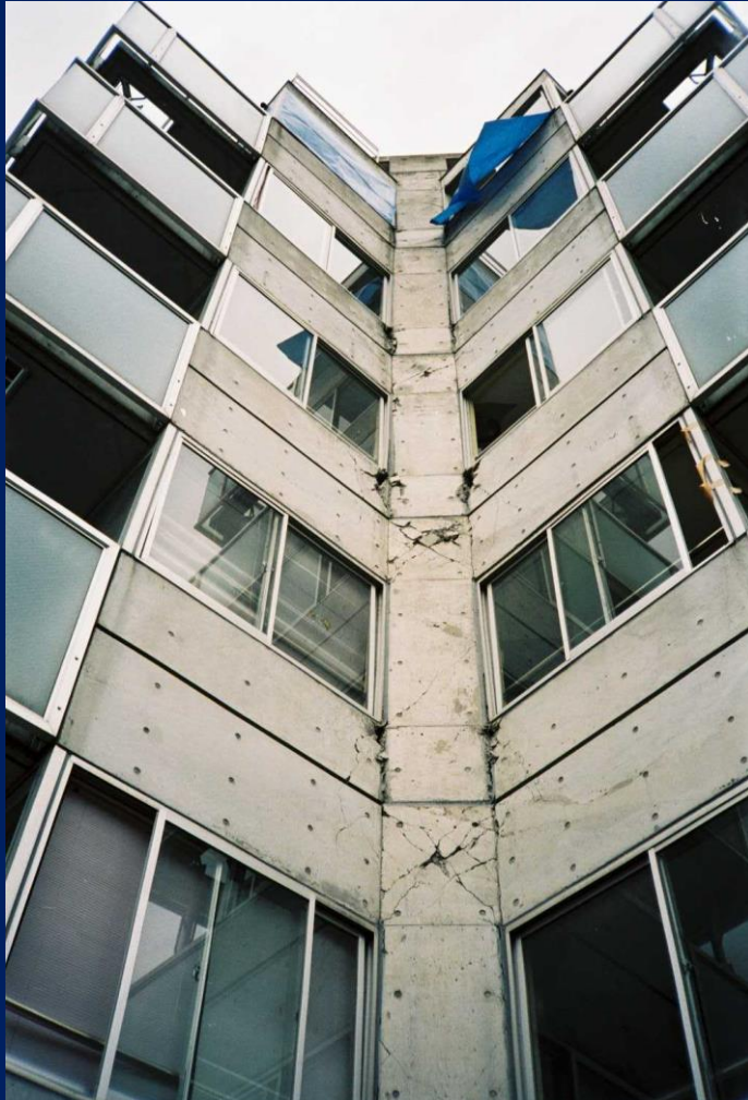
Cracks of Beam Column Joint (New Code)
