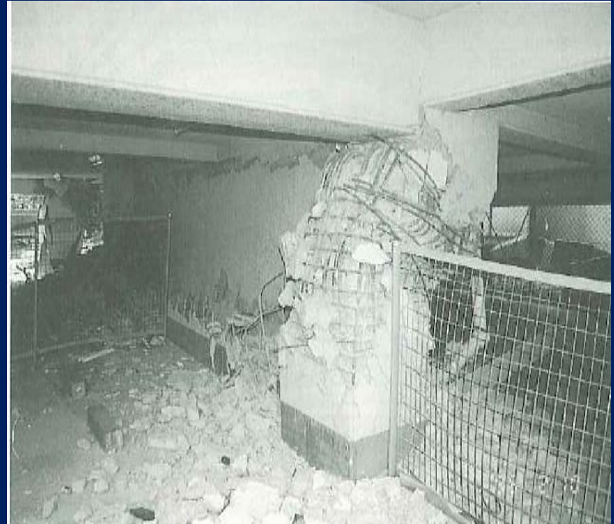
Failure of First Story (New Code)
