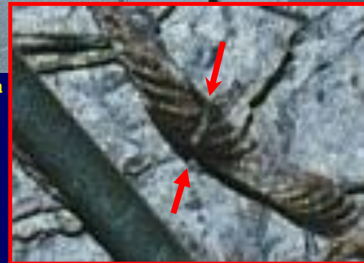
Breaking of rebar
