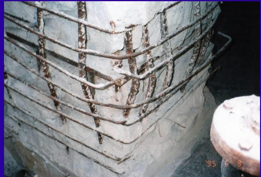
Taking off of damaged concrete portion
