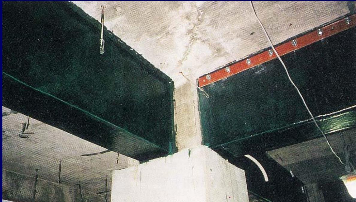
Beam retrofit by carbon fiber sheet
