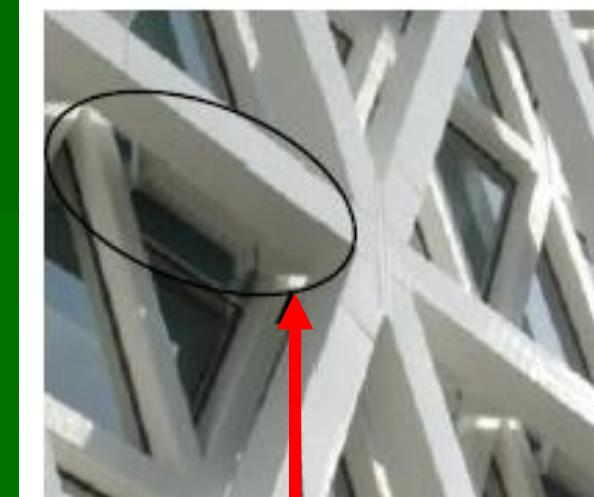
Joint of triangle frame and top bracket
