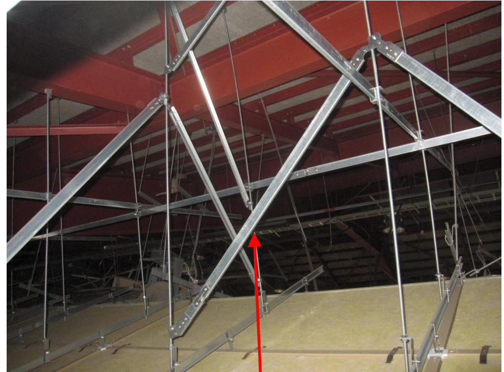
The fixed parts after 2008 EQ escaped damage
