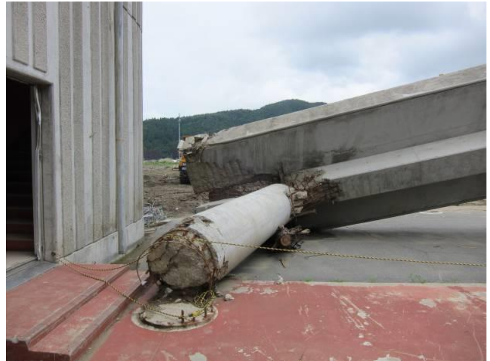
Bottom of column of passage.
