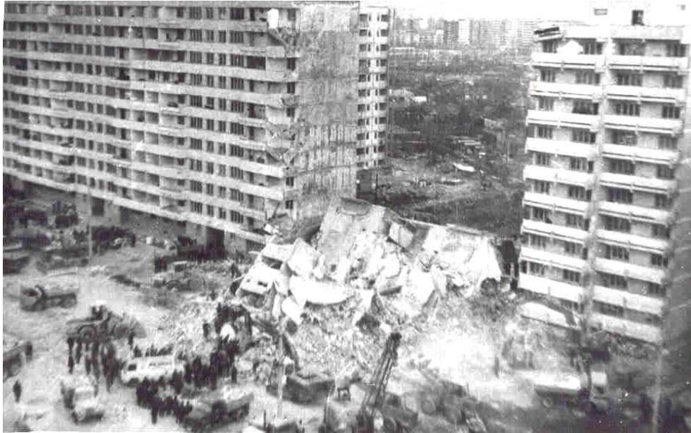
Partial collapse of a section in Bloc OD16, Bd. Pacii No 7, Bucharest, built in 1974
