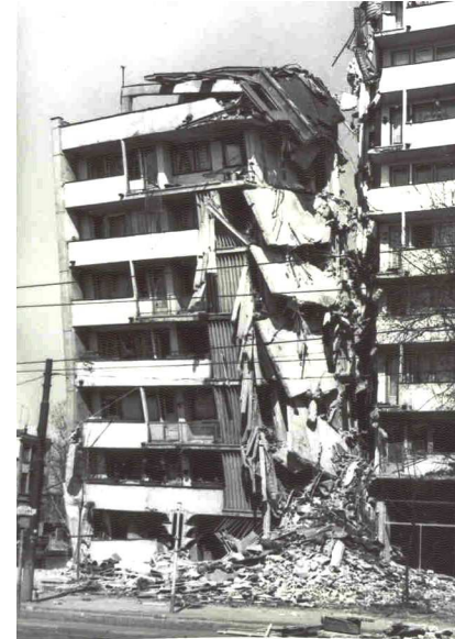
Partial soft-story type collapse of Bloc 30 “Lizeanu”, Stefan cel Mare Street, No. 33, Bucharest, built in 1962
